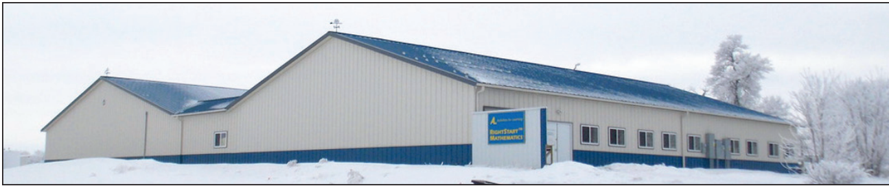
The new addition to Activities for Learning, Inc., which recently expanded to more than double its original size, is on the left.
